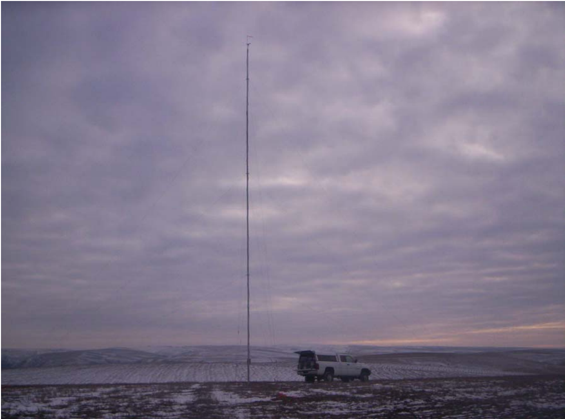
Appendix B: Photograph of the 20 meter tower placed on Fulton Ridge.
